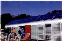
The University of Puerto Rico team's fundamental design for 2002 is based on the use of passive solar technologies. The students believe that it's also important to achieve a very efficient spatial solution that feels comfortable and looks attractive. They wanted to design a house that goes beyond merely incorporating existing solar energy technologies—a house that can actually influence lifestyles and make an impact on the way we humans understand and relate to our space, our planet, and our sun.
